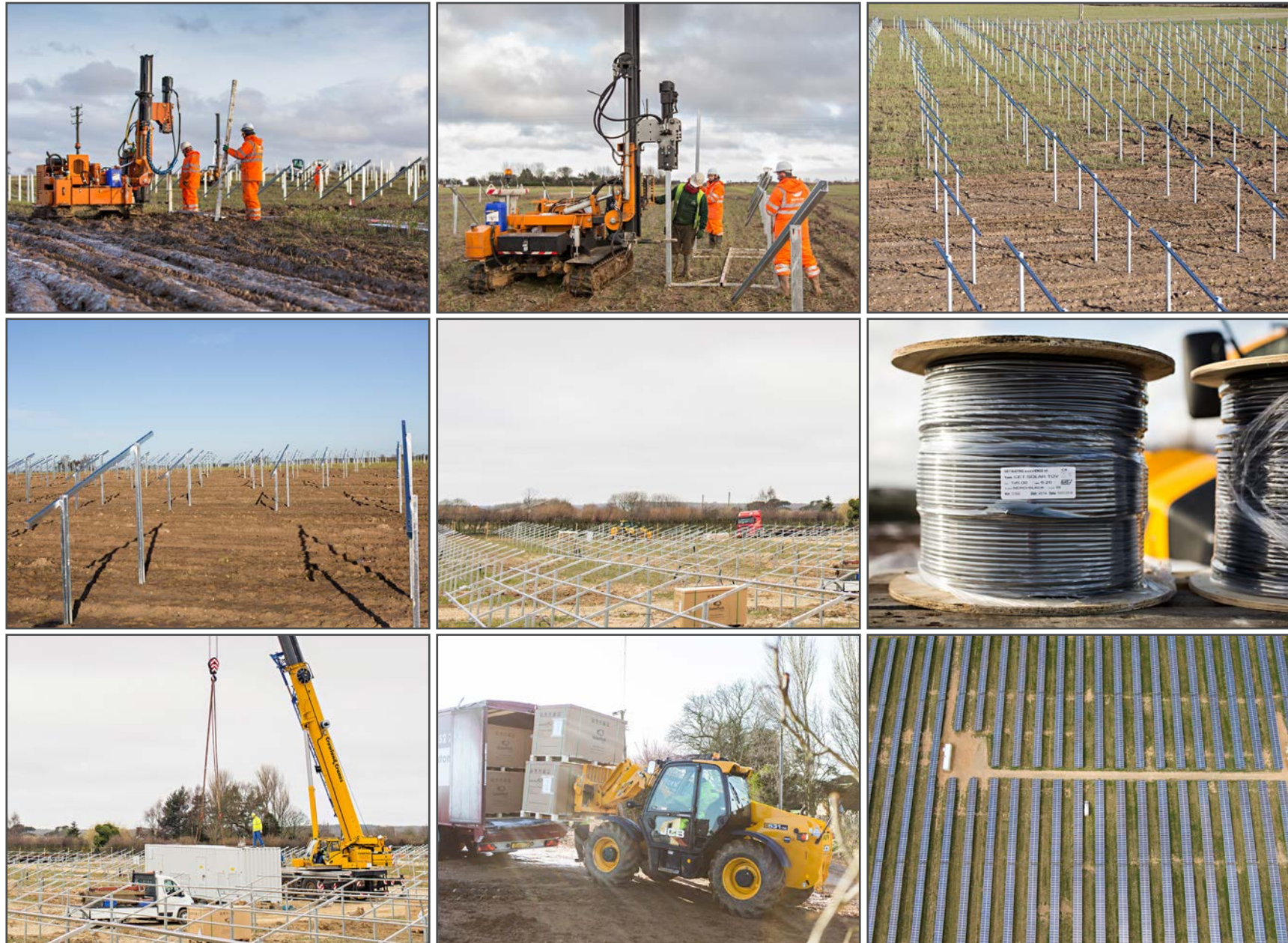
Plate A.4 - Photographic Sequence of Construction Process
