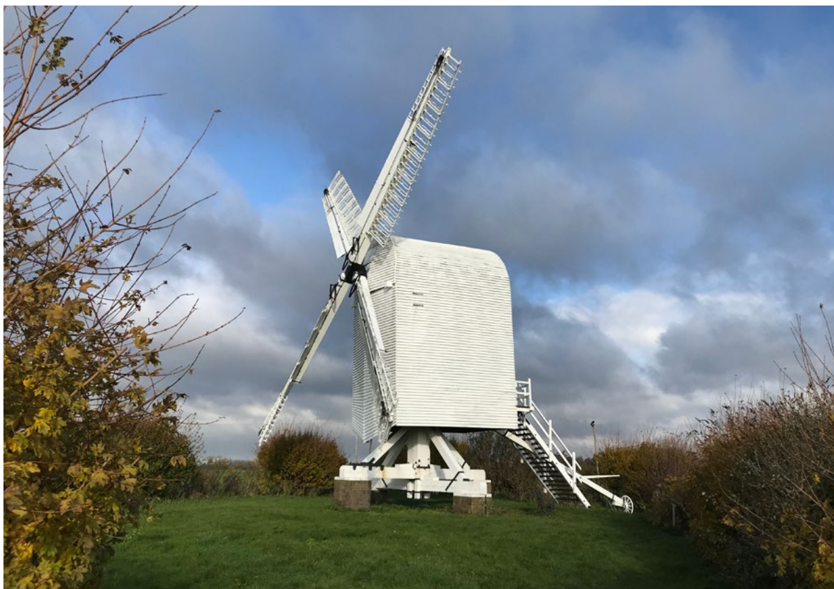
Figure 7 Chillenden mill after restoration.
