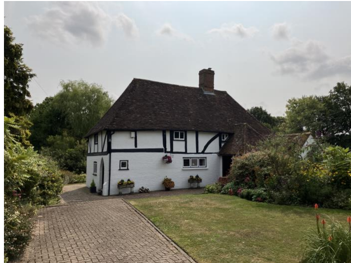
Figure 1. Possingham Farmhouse from drive (looking SE)
