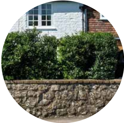
RAGSTONE ON WALLS
