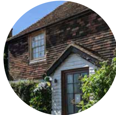
TILES ON THE FACADE
