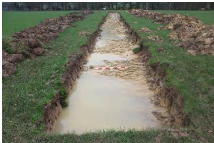
Trench 122, Facing East
