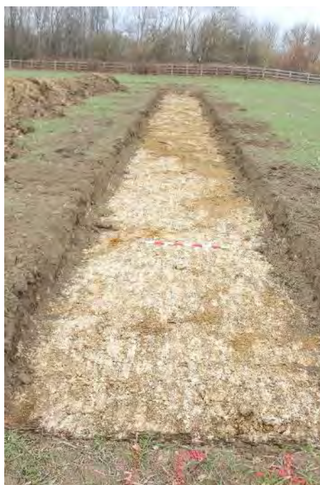
Trench 3, Facing North
