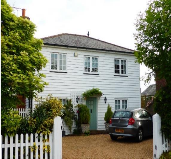
White Gates (left) is an example of an infill property which employs the local built form and materials.
