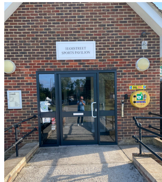
Hamstreet Pavilions new front door.
