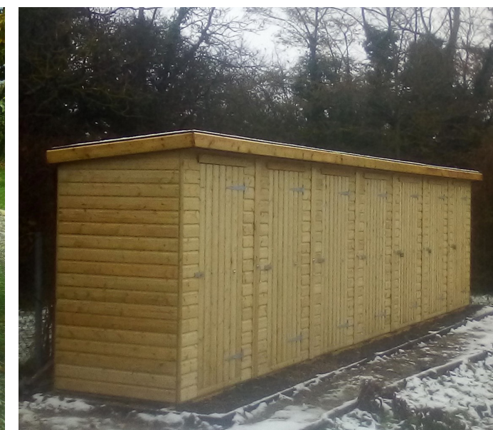
New bespoke tool shed for the tenants of Aldington Meadows allotments.
