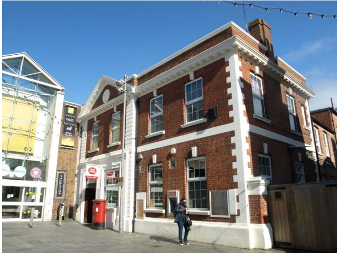
The County Square development truncates the symmetry of the post office building
