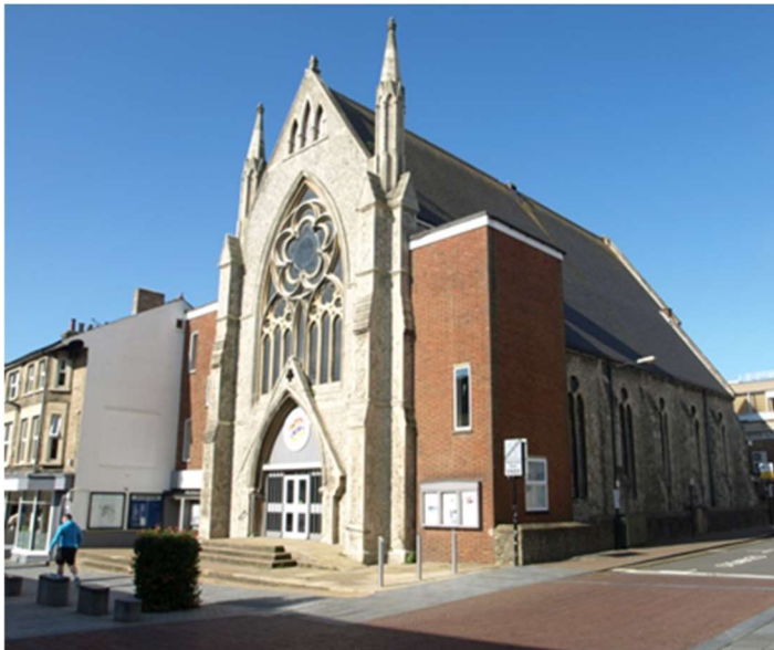
Despite the unfortunate flat roofed brick side extensions and the slight recess from the general street frontages, the contrasting scale, use of ragstone (reminiscent of St Mary's church) and prominent location set above steps at the centre of Bank Street within a wide paved apron, Centrepiece Church is a prominent notable local building.
