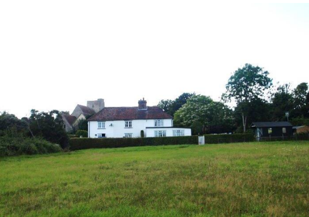
The cottages face onto, and are prominent in views from, the open countryside to the north east and can be seen in the same view with the church tower (right). The buildings and gardens also abut the public footpath running south west back past the church. Whilst not listed buildings, the white weather boarding and prominent location make these notable local buildings in terms of the character of this part of the Conservation Area and in understanding the historic evolution of the village.
