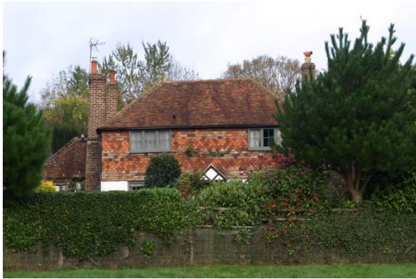
The listed Piran (now Candlemass) Cottage (left) comprises two parallel ranges. The south range is refaced with red brick now painted on the ground floor and tile-hung above whilst the north range is a C19 addition, with its first floor oversailing in imitation of timber-framing. The cottage has a hipped tiled roof with chimneys and is located within a neat hedged landscaped garden adjoining the footpath and church yard.
