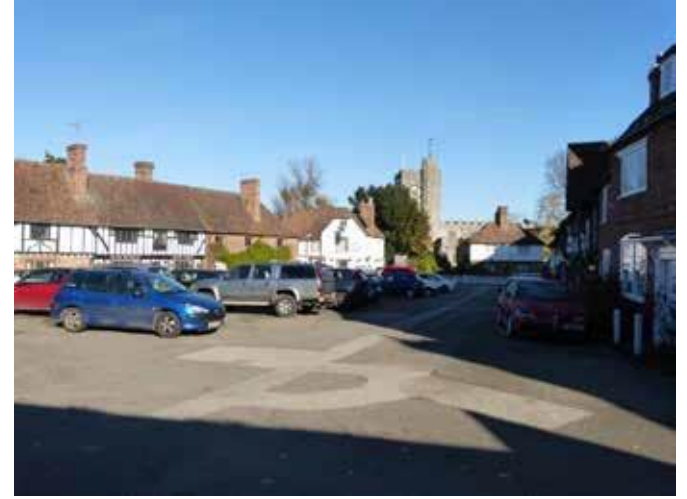
Resurfacing required in The Square
